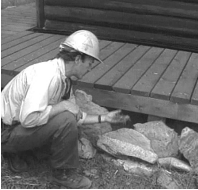
FIGURE A.17.1.8.3(a) Leaf Litter and Needles Collect in Small Spaces. (Courtesy of Firewise Communities Program.) [1144:Figure A.4.2.4.3(a)]
